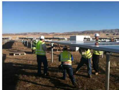
CVSR workers install panels on the project site
